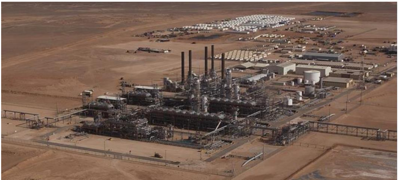
Figure 2. The In Salah site (Algeria). Picture courtesy of Equinor.
