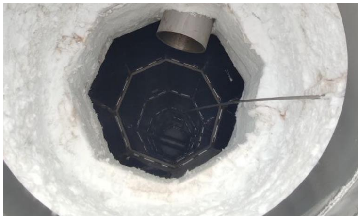
Figure 11: Reactor interior status.
