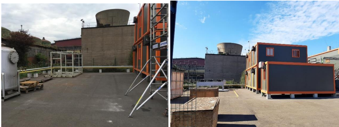
Figure 2: Construction site of the pilot plant
