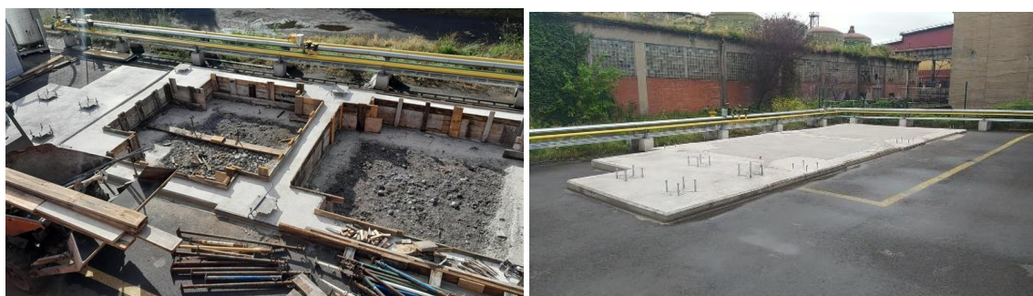
Figure 3: CASOH pilot plant foundations
