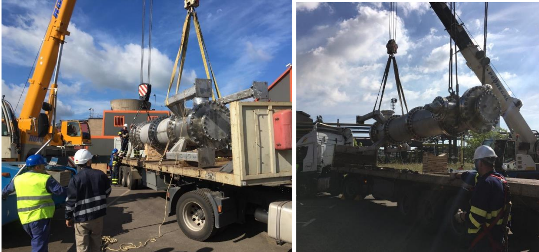
Figure 10: Reactor lifting and placing maneuver
